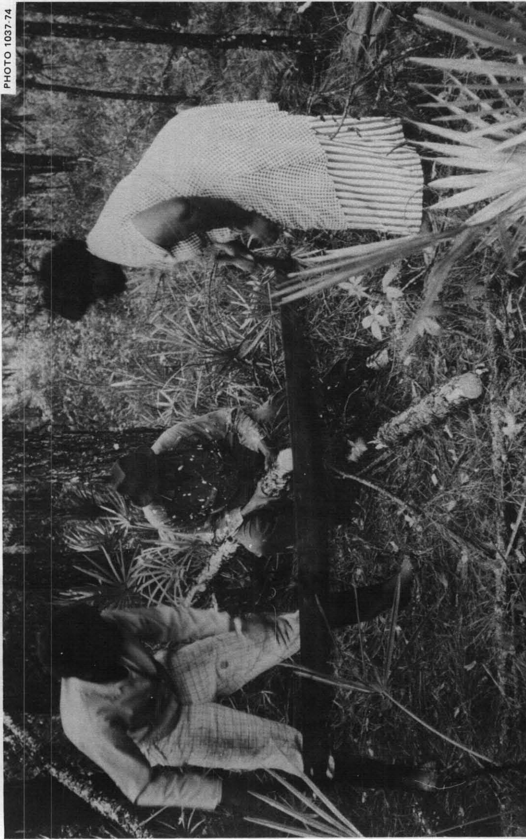
Fig. 5.15. Cutting a small felled tree into one of the specified lengths needed to build pole cribs. Later the cribs were lined with bed sheets and then filled with earth. Instead of following the instructions and pulling long poles to the shelter-building site, where they should have been cut to the desired lengths, this family chose to have the children carry small poles one at a time to the site.
